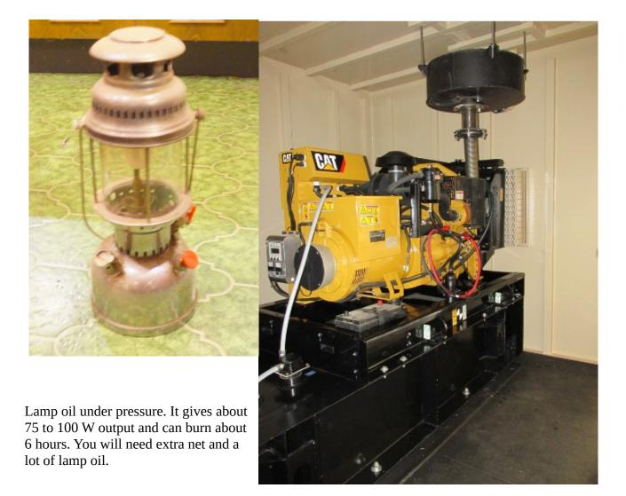
Generator in an iron shelter. External wire are first connected after a HEMP or during normal blackout. Even the starter battery is not connected although we are in an iron shelter. It may be worth investigate I such a generator, if you are floating with money. END
